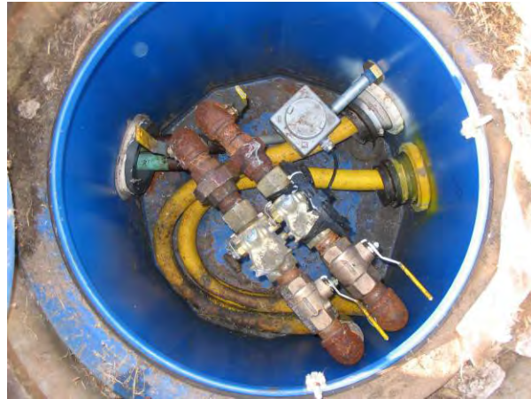
Figure 20. Image of sump with product residue.
